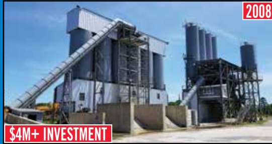
STANDLEY Concrete Batch Plant
