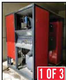
(3) KRAFT CURING Direct-fired Vapor Generators
